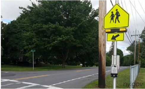
Rectangular rapid flashing beacon
