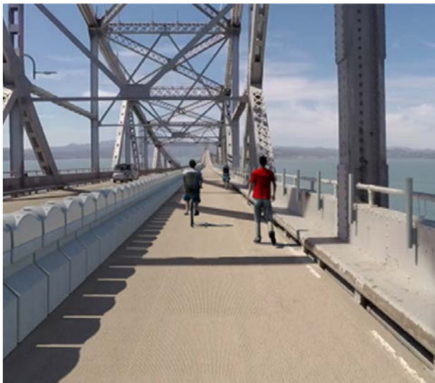
Multi-use trail on bridge.
