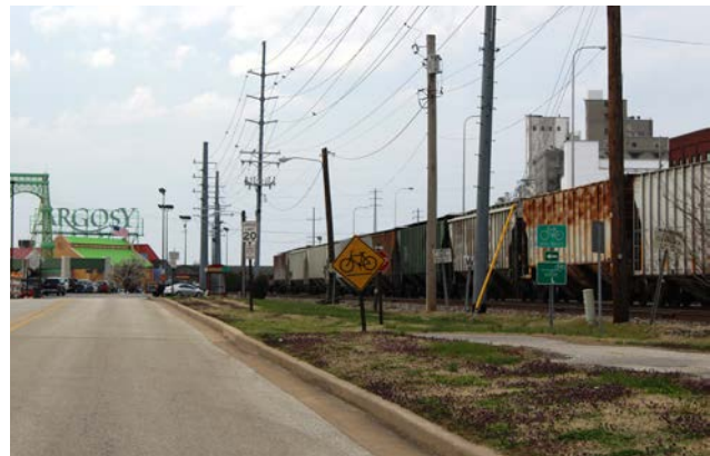
End of Confluence Trail in Riverfront Park, near casino.
