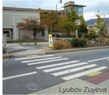
Refuge island in median
