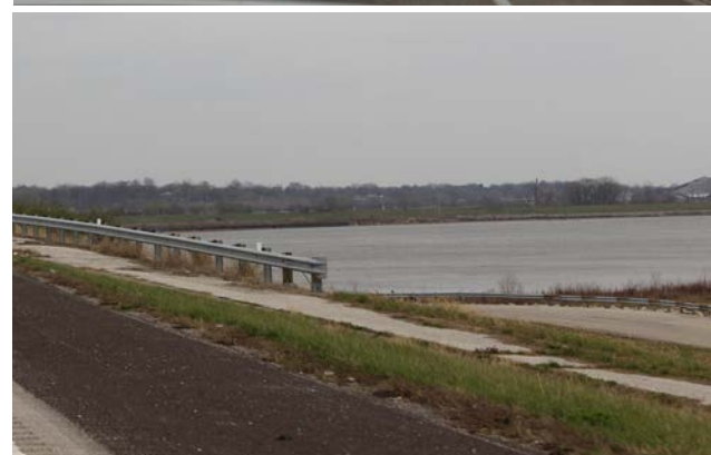
Top: Faded bike lanes on Clark Bridge. Bottom: Bike access ramp on Missouri side of bridge.
