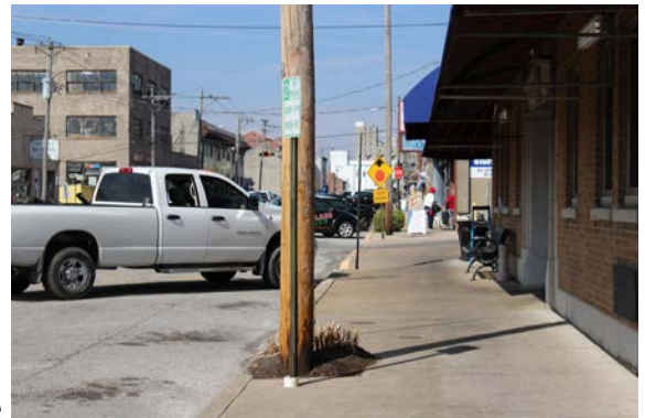
Broadway sidewalks, utilities in pedestrian zone.
