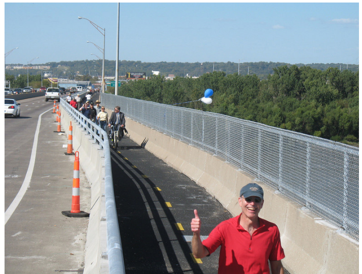
Multi-use trail adjacent to highway in Kansas City.
