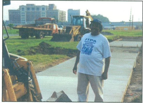
Trail construction in East St. Louis, Illinois
