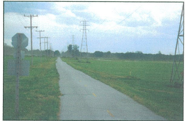
The Madison County Transit Nature Trail near Pontoon Beach, Illinois.
