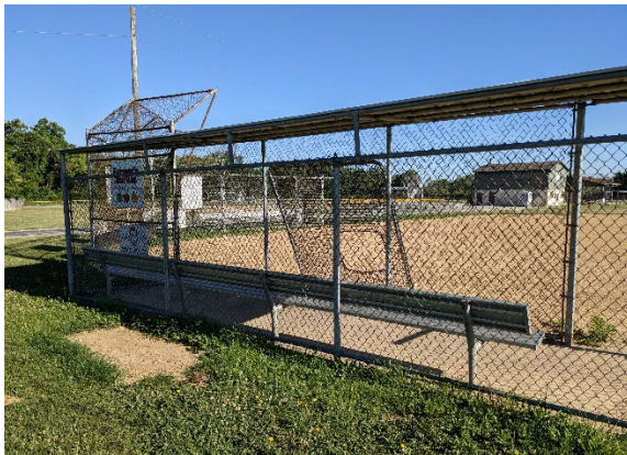
Approximately 3 fields have been kept in playable condition.
