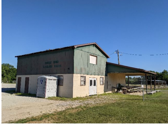
Existing concessions, restroom, and maintenance building. Restrooms are small and not ADA compatible.
