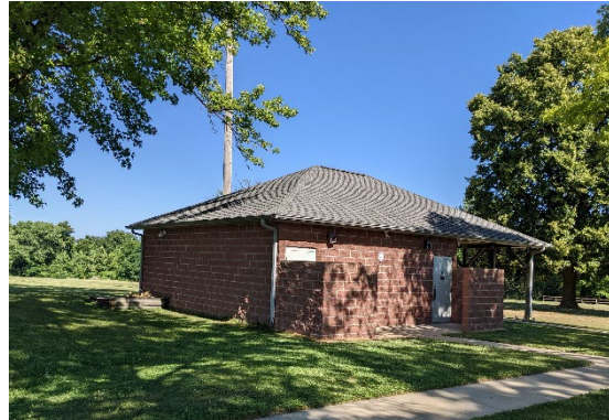
Concrete block restroom facility.
