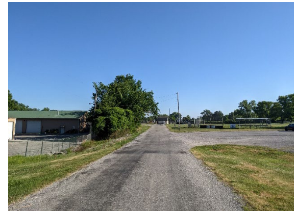
Entrance drive is narrow at ~17' wide and no shoulder on the west side.
