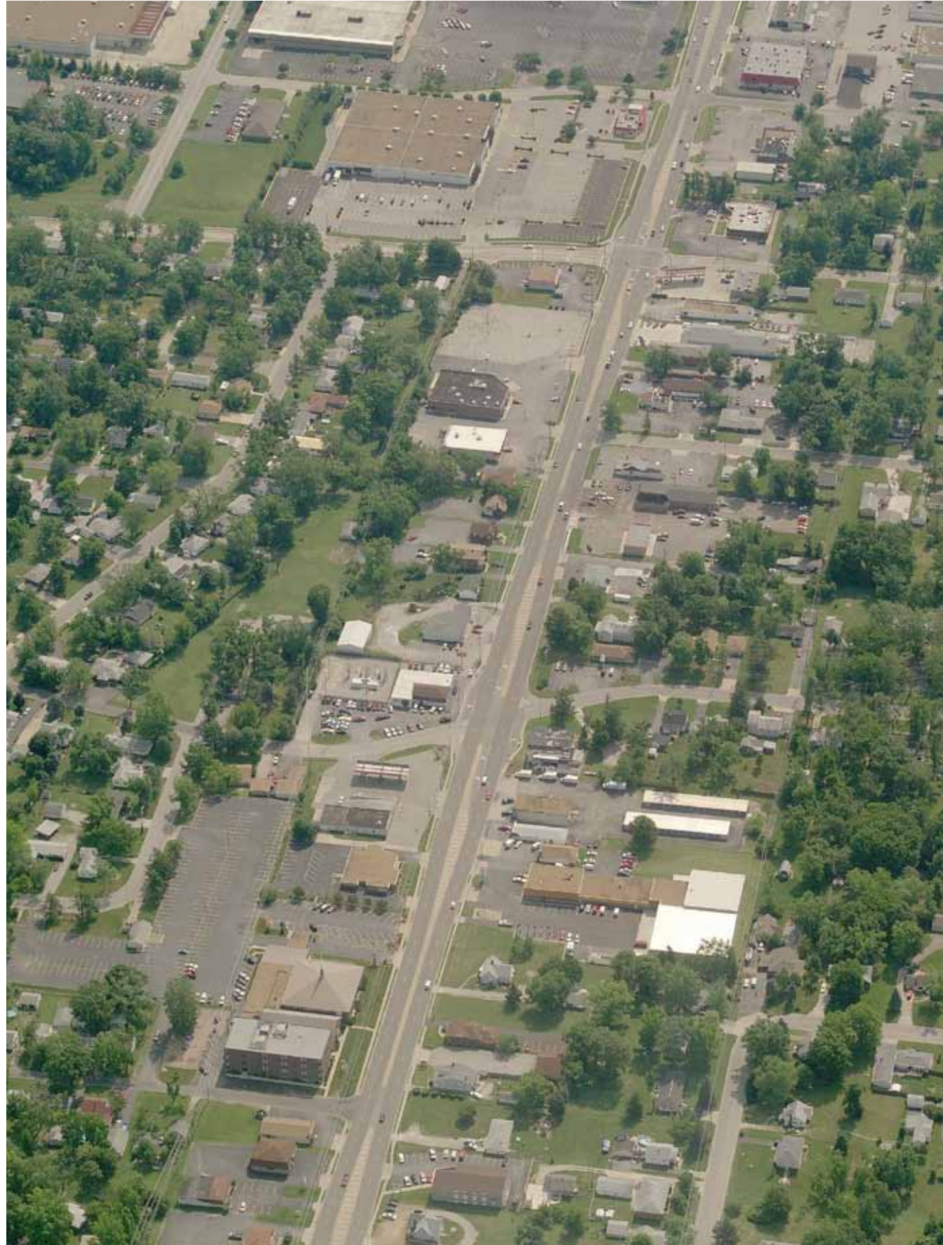
Lincoln Highway (from the west)
