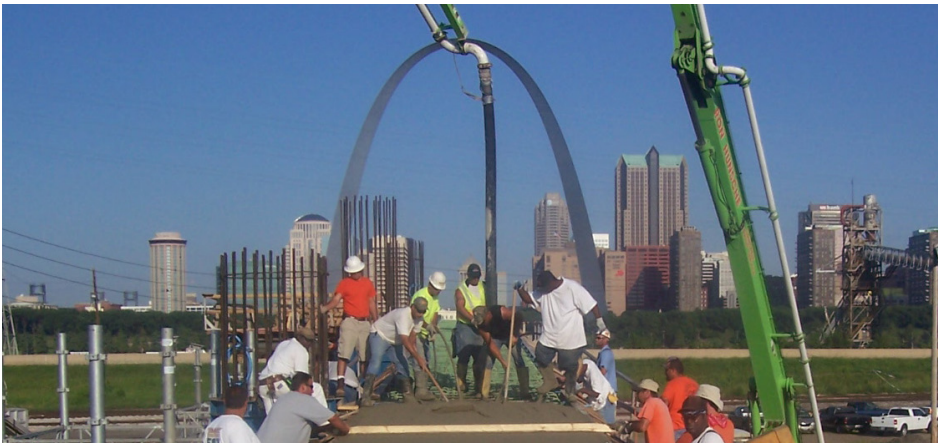
Construction of the Mississippi River Overlook at Malcolm W. Martin Memorial Park, East St. Louis, IL.
